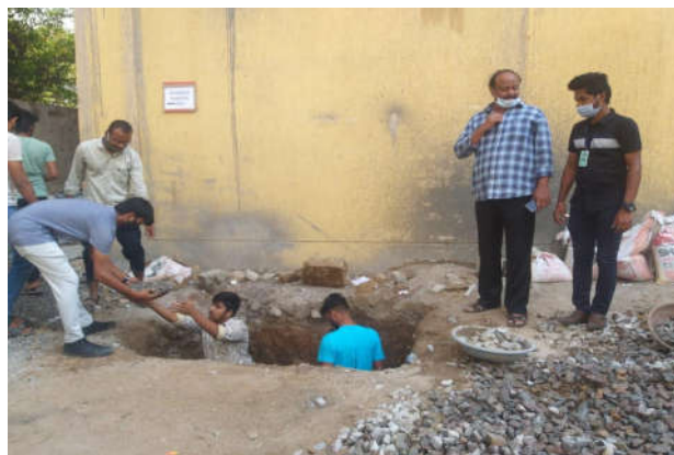
Figure 1 Construction of RWH pit at BJR College
